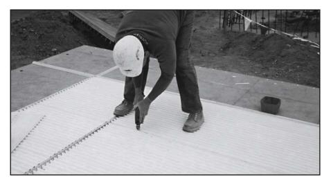
Self-drilling and tapping, the flat head fits flush with the liner, and may be used for steel or wood forms. A screw gun with adjustable torque setting is also recommended.
